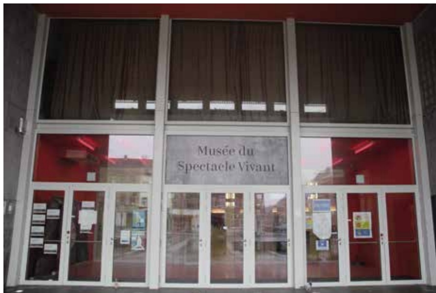
Façade de Central © C. Callico
